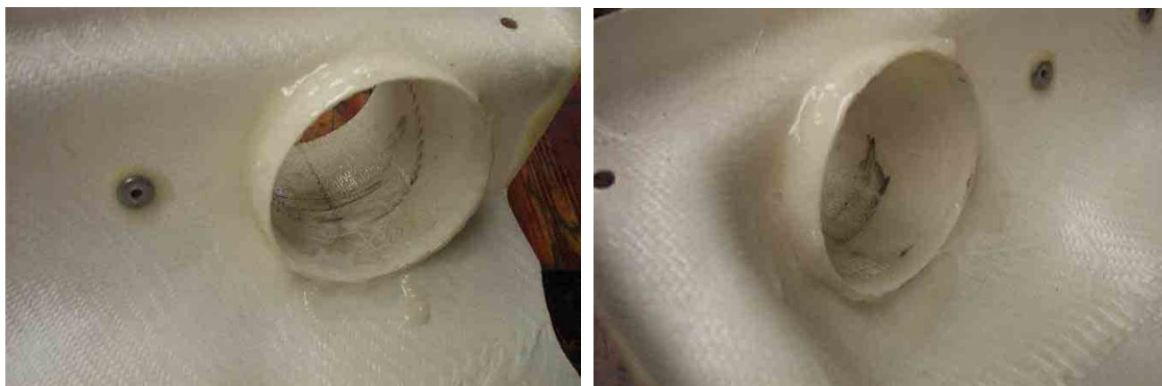
Figure 36. Air Filter Box Plumbing – Incorrect
